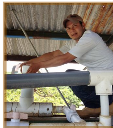
CTI: A field technician checks on a chlorinator in rural Nicaragua
