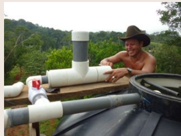
AN INSTALLED CHLORINATOR IN NICARAGUA
